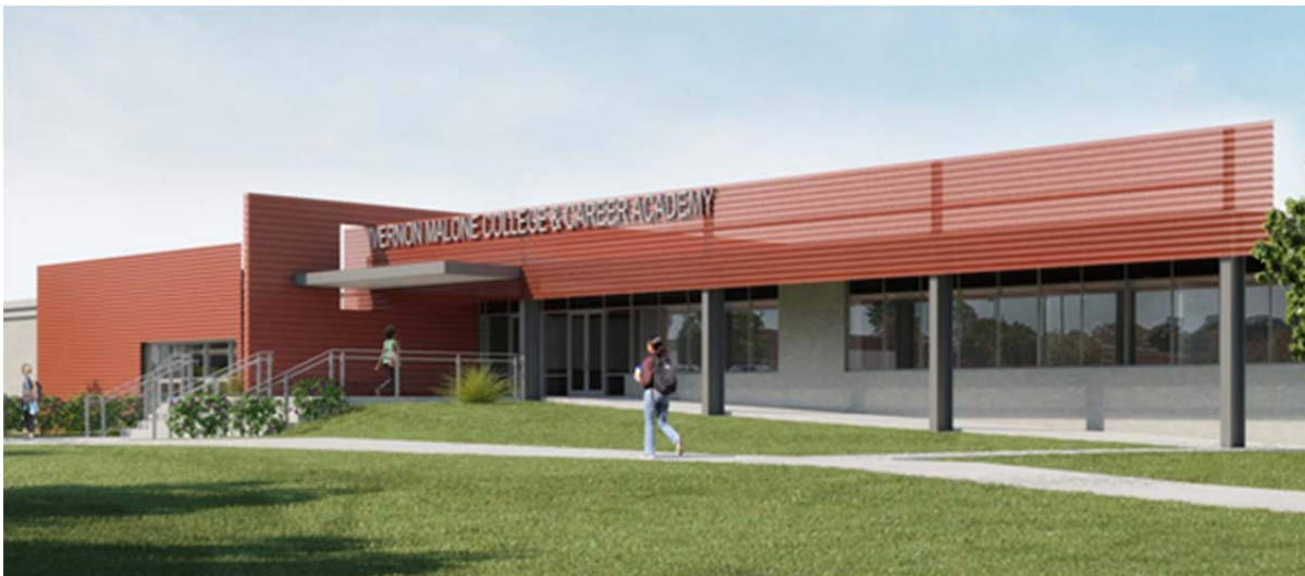
Vernon Malone College and Career Academy, 2200 South Wilmington Street Raleigh, North Carolina
